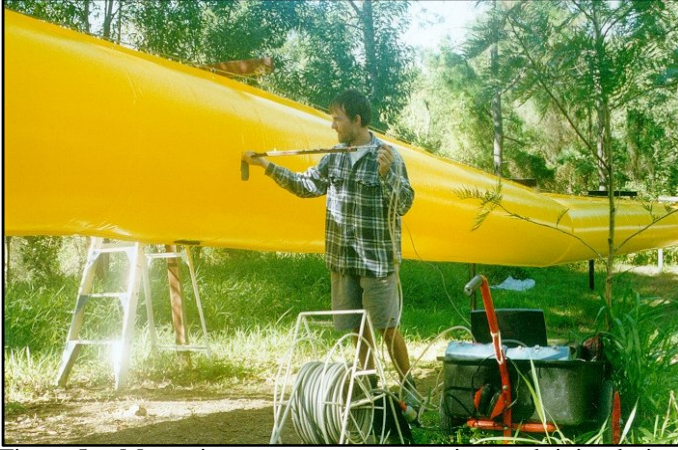
Figure 5. Measuring apparatus, suspension and joint during duct leakage measurements.
