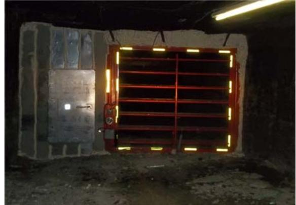
Figure 8. Louvered Regulator Installation
