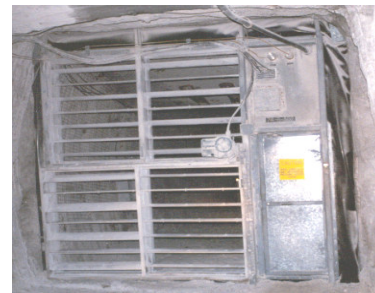
Figure 7 An example of a louvre regulator.
