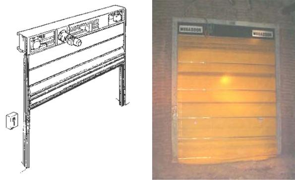
Figure 9 Schematic and photographic views of a roller door regulator
