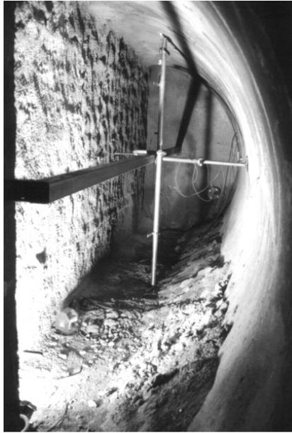
Figure 7. Internal view from the explosion side of the 325 mm thick Trecete Seal.
