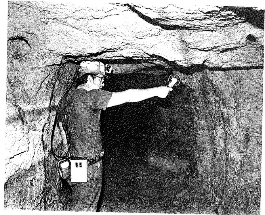
Figure 6. Vane anemometer measuring air velocity.
